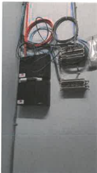
Floor 7 Riser unmarked fiber panels
